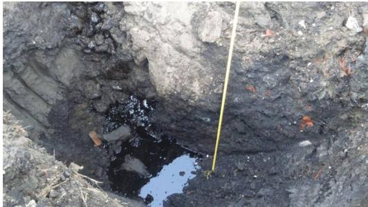
There were several „surprises” during the work. Trying to built an infiltration well, a former drain was found f oil! The drain will be washed through by a pair of infiltration wells.
