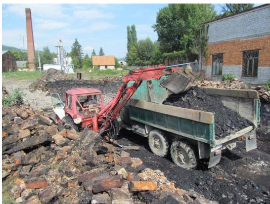
Main contamination source – the half underground mazout reservoir - still could not be fully demounted. This problem is partly solved, the solid wood resin is taken out, the concrete and walls are cleaned. Drain will be constructed in the middle.
