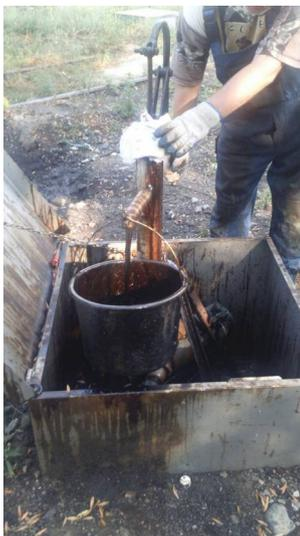
Most difficult handy work is skimming the free phase floating material. Temporarily it was solved by a handy pump.
