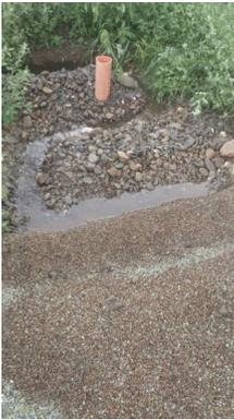
There are black manganese particles in cleaned water. We tried an experimental post-cleaner with zeolite filter that was only partly successful. A bigger post-filtering reservoir is needed.
